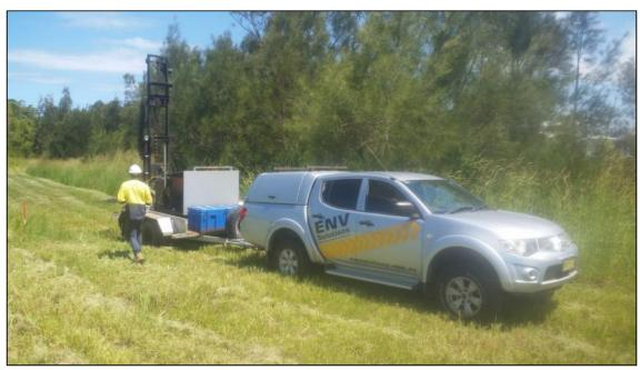
Plate 5: Setting up to drill at one of the boreholes along the site's western boundary.
